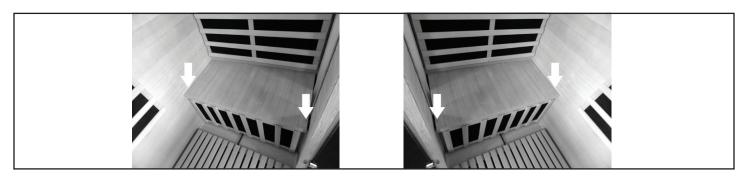
8. Lift the ROOF above the sauna, feeding the control panel and heater cables through the corresponding holes. Feed the cables for the AM/FM CD PLAYER through the hole in the bottom of the ROOF. Secure the ROOF to the sauna with 1-1/8" SCREWS. Connect the control panel and heater plugs.
