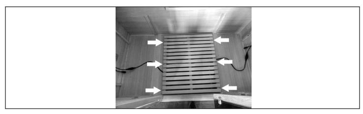
6. Slide each BENCH HEATER PANEL into place between the FRONT and BACK PANELS. Connect the heater plugs. *Note: Make sure each FLOOR HEATER cable is placed through the groove in the bottom of the corresponding BENCH HEATER PANEL*.
